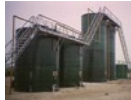
Oil storage tanks
