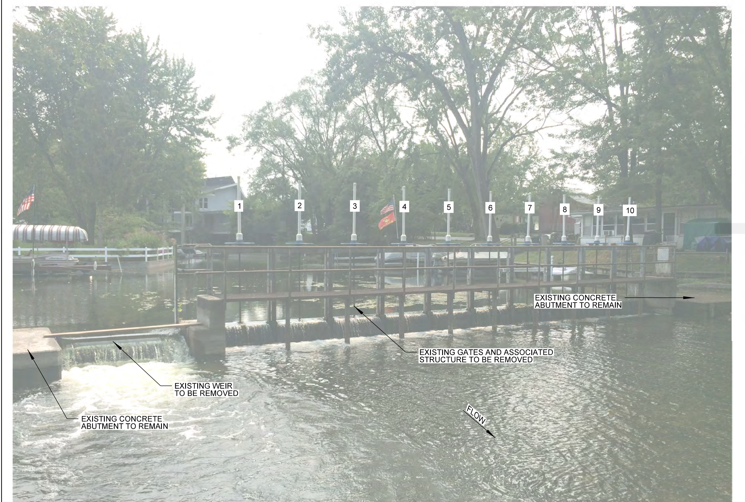
Photo taken from downstream looking northeast (upstream).
