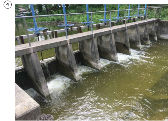
EXISTING OUTLET STRUCTURE LOOKING UPSTREAM
