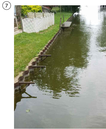
EXISTING UPSTREAM SHEET PILING
