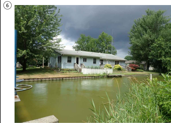
EXISTING UPSTREAM SHEET PILING
