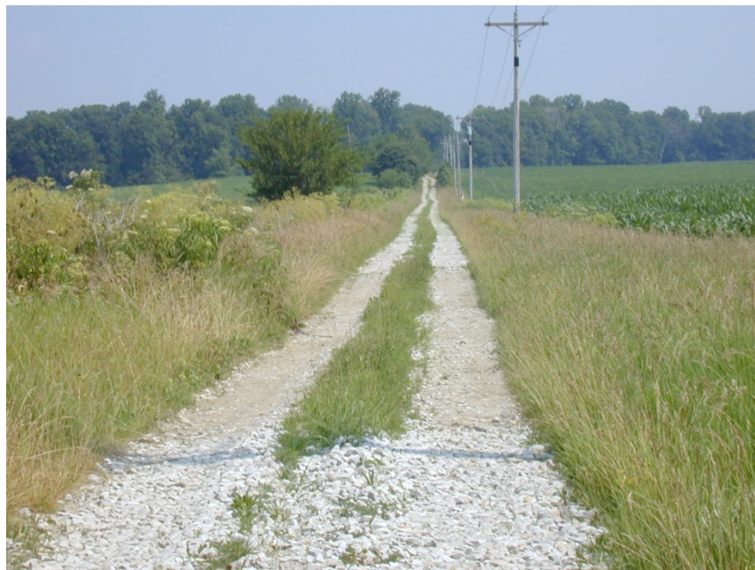
Permanent haul road protected by rock.
