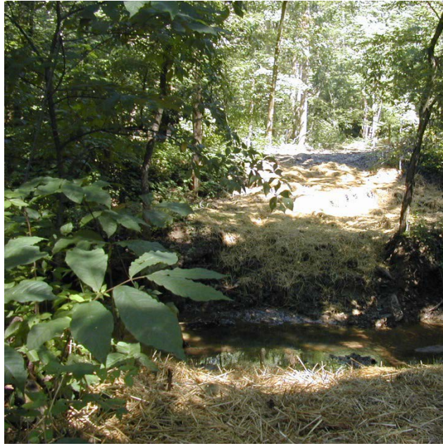
A well-closed-out stream crossing, with seed and straw applied to stabilize bare soil and promote re-vegetation.
