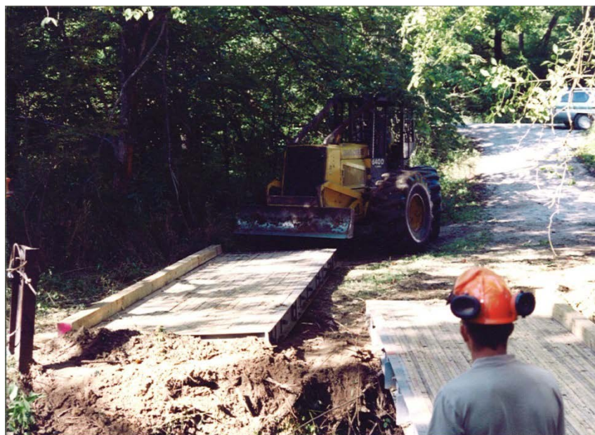
Dozer installing bridge for stream crossing on timber harvest site.
