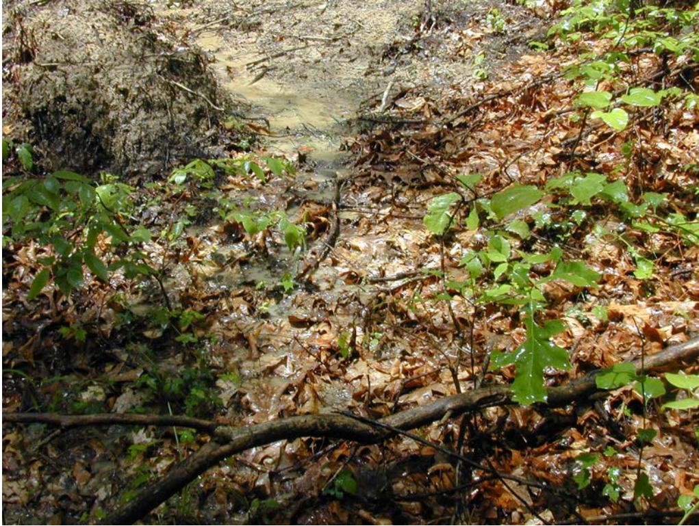
Water bar outlet conveying runoff On to the stable forest floor.
