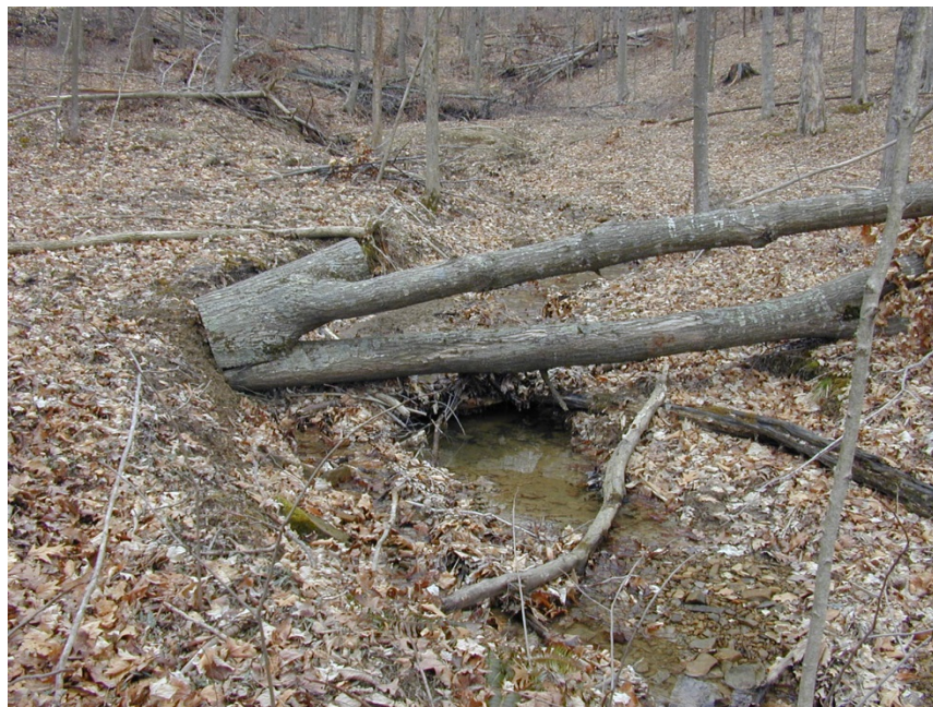
Logging debris in streams can obstruct stream flow, leading to the stream carving a new bank, which results in erosion and sedimentation going directly into the stream.
