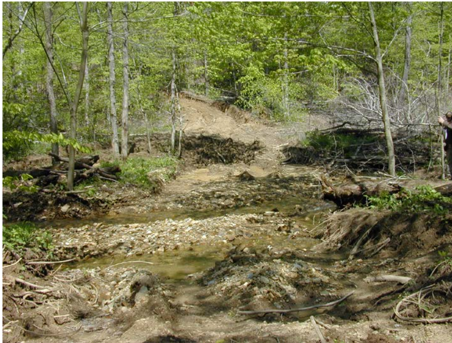
Poorly executed and stream crossing not closed out after harvest completed.
