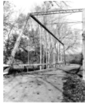
Smith Bridge Company, Toledo OH: 2 remaining
