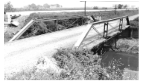
Two bridges from the same county: a 1900 Pratt pony (Above) and a 1917 Warren pony (below)
