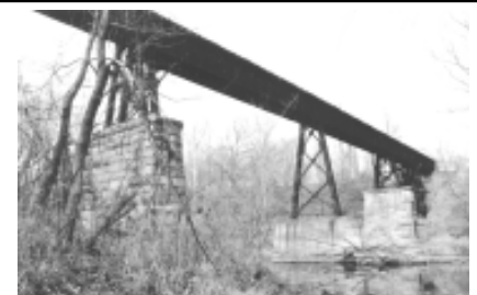
This plate girder viaduct is one of Indiana's longest and highest spans.
