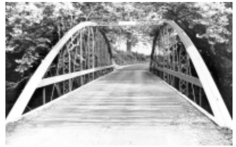
This 1870s Bowstring Arch truss represents the early days of metal bridge construction in Indiana.
