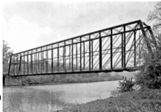
Laughery Creek Bridge (1878) in Dearborn County
