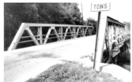
Warren pony trusses (above) are fairly common in Indiana; Warren deck trusses (below) are not. Fewer than 10 Warren decks remain today.
