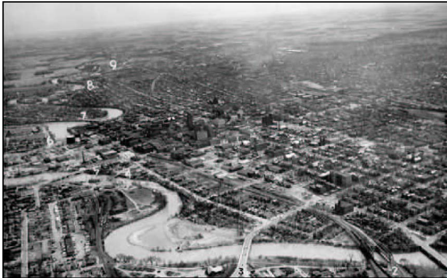
Figure 7. Photograph of Fort Wayne showing flooding along the St. Marys River in the 1940s (ACPL Community Album 2005b).
