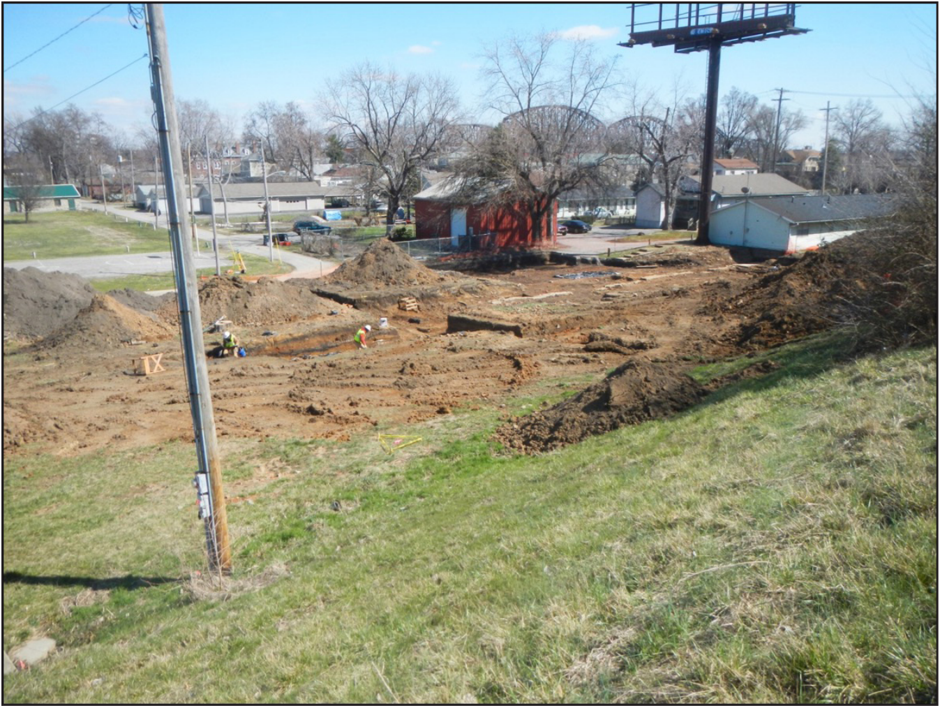
Figure 3. Overview of data recovery excavations in progress, facing southeast (Cupka Head 2015:23).
