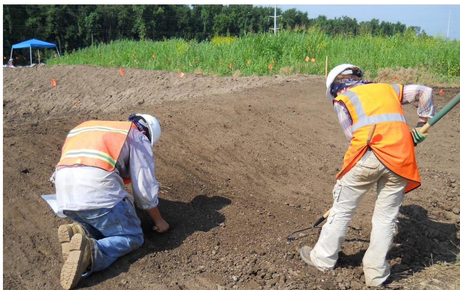
Figure 4. Recovery Phase, North Berm exterior, showing hand excavation with rake and trowel (the former location of the barn is the grass-covered area).
