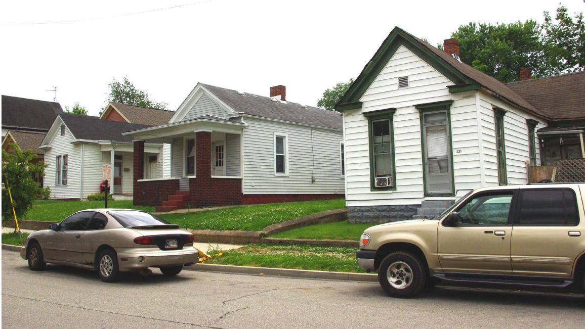
East Spring Street H.D. Boundary Increase. Amendment, and Additional Documentation Floyd County, IN Photo #0019
