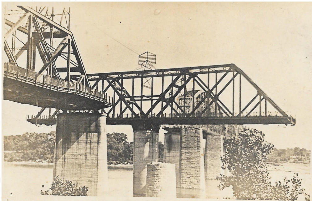
East Spring Street Boundary Increase, New Albany, Floyd County, Indiana K & I bridge with swing span open for river traffic.
