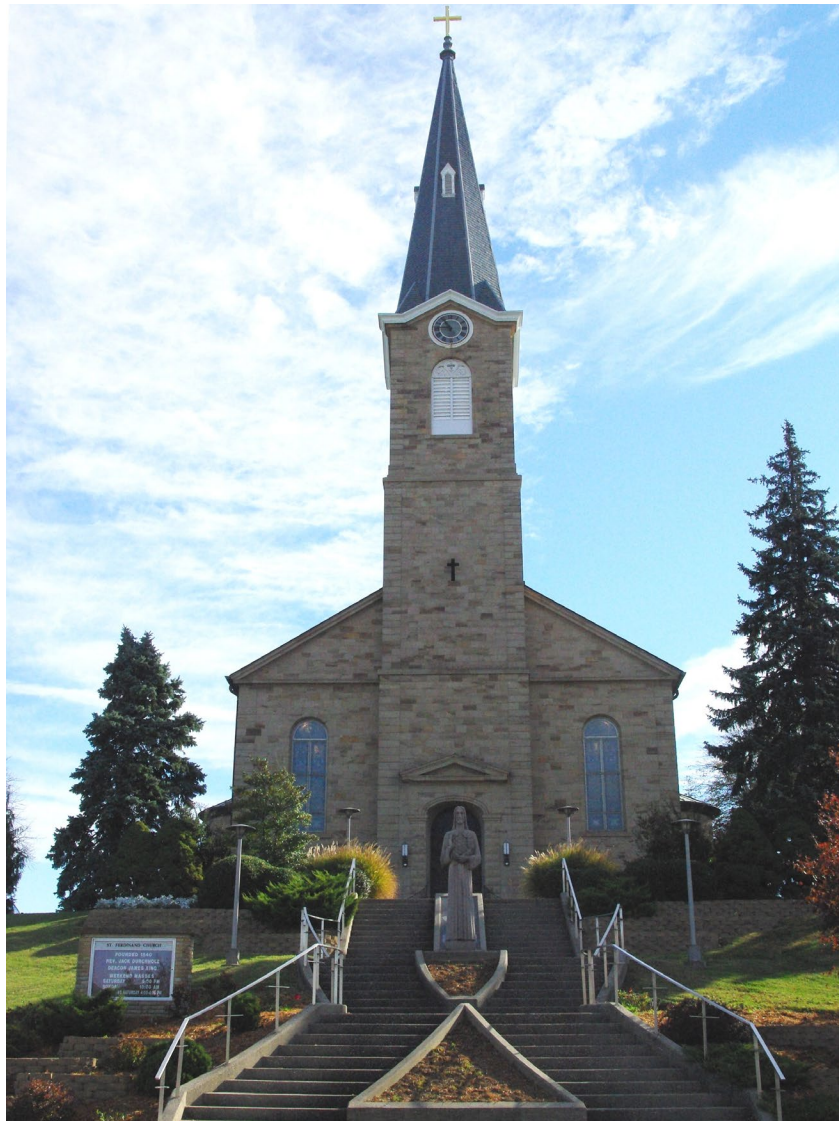
St. Ferdinand Parish Historic District, Dubois County Photo 0004
