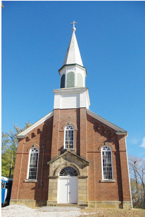
St. Ferdinand Parish Historic District, Dubois County Photo 0017
