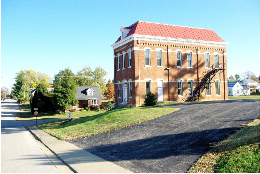
St. Ferdinand Parish Historic District, Dubois County Photo 0003
