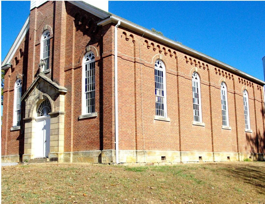
St. Ferdinand Parish Historic District, Dubois County Photo 0018
