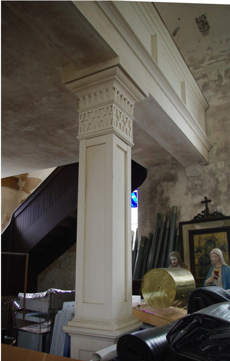
St. Ferdinand Parish Historic District, Dubois County Photo 0022
