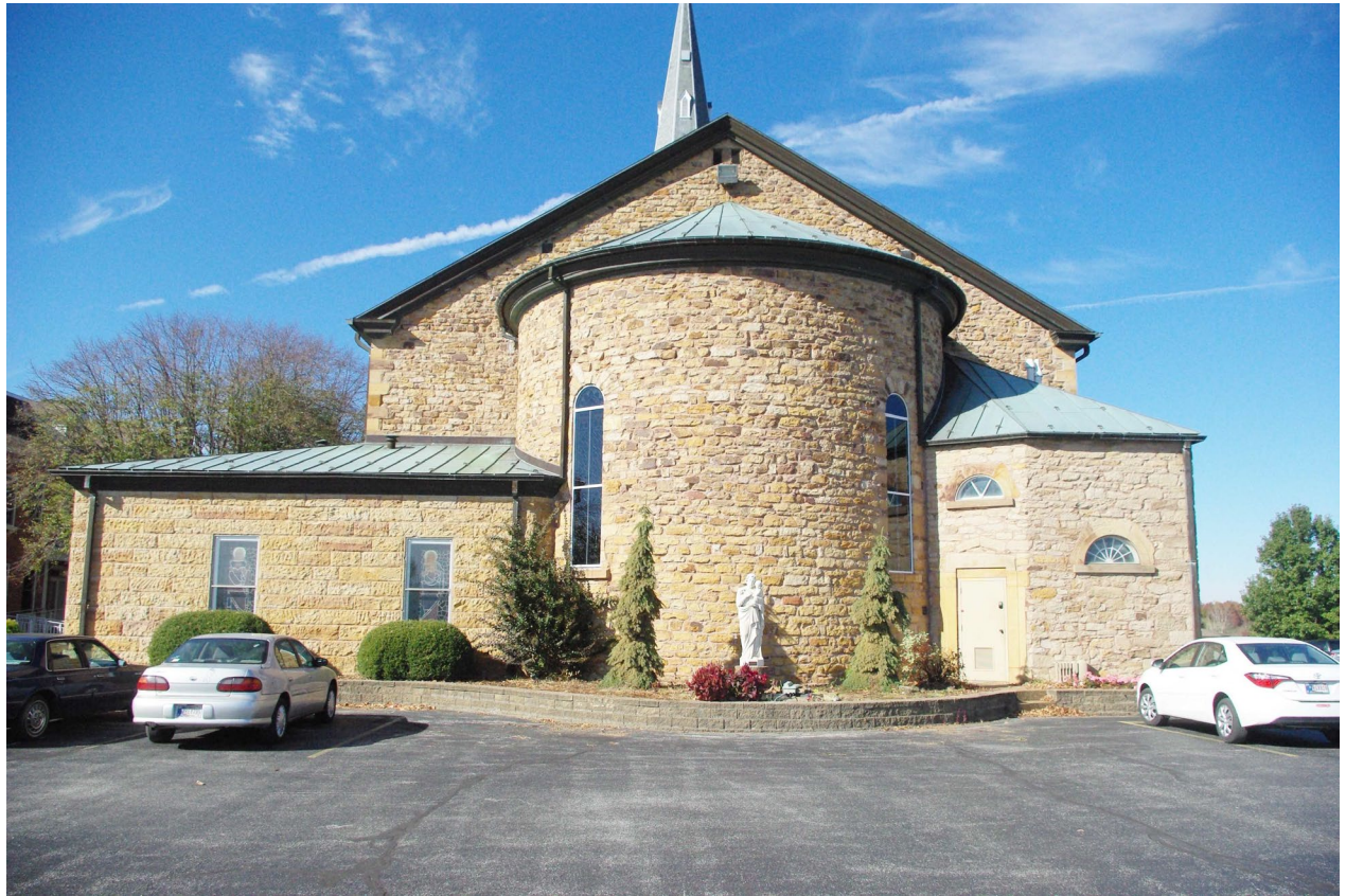
St. Ferdinand Parish Historic District, Dubois County Photo 0011
