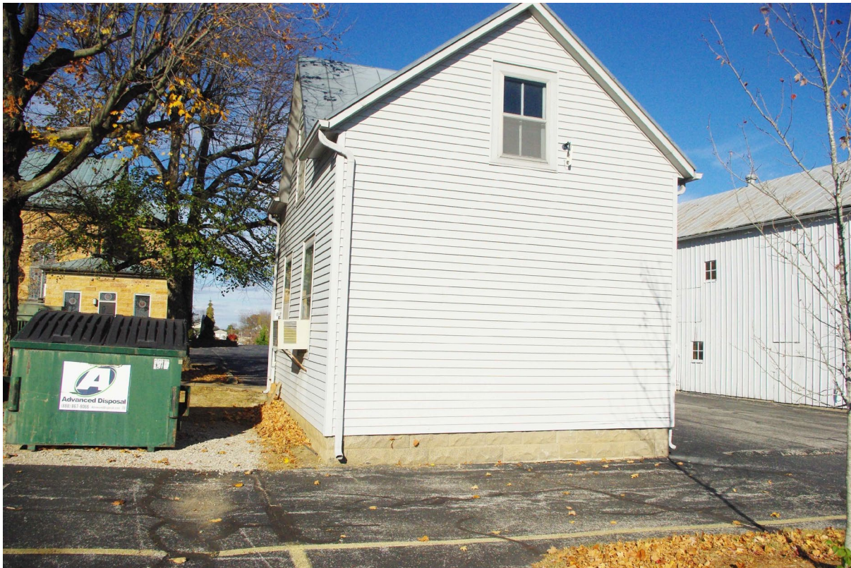
St. Ferdinand Parish Historic District, Dubois County Photo 0009
