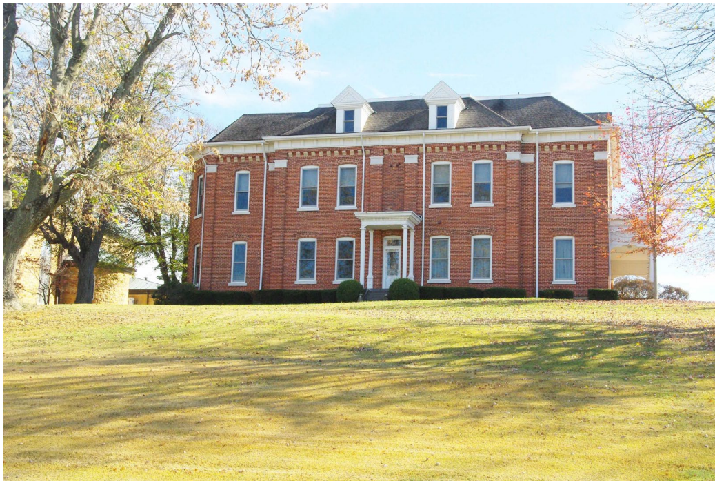
St. Ferdinand Parish Historic District, Dubois County Photo 0007
