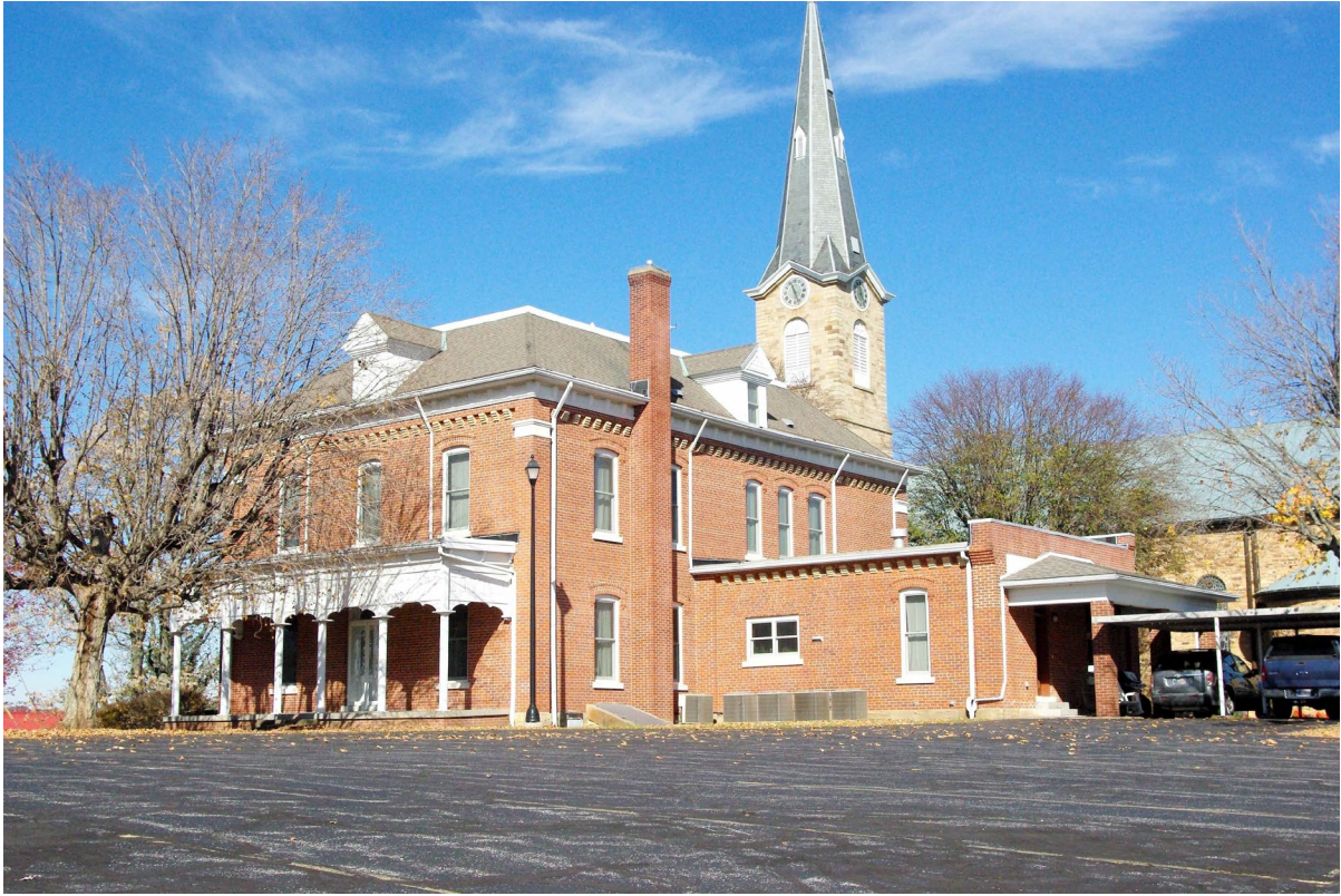
St. Ferdinand Parish Historic District, Dubois County Photo 0008
