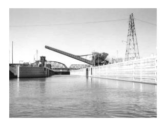
Locks - A man-made "water elevator" built on a canal and used to raise and lower boats to different levels. The McAlpine Locks on the Portland Canal at Louisville are one of 21 locks in the Ohio River System (see above).
