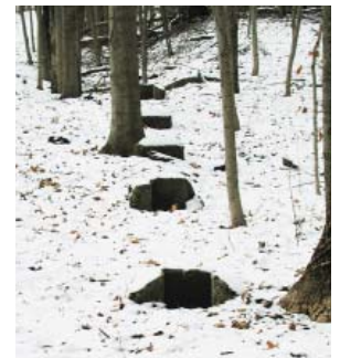
Interurban station foundations
