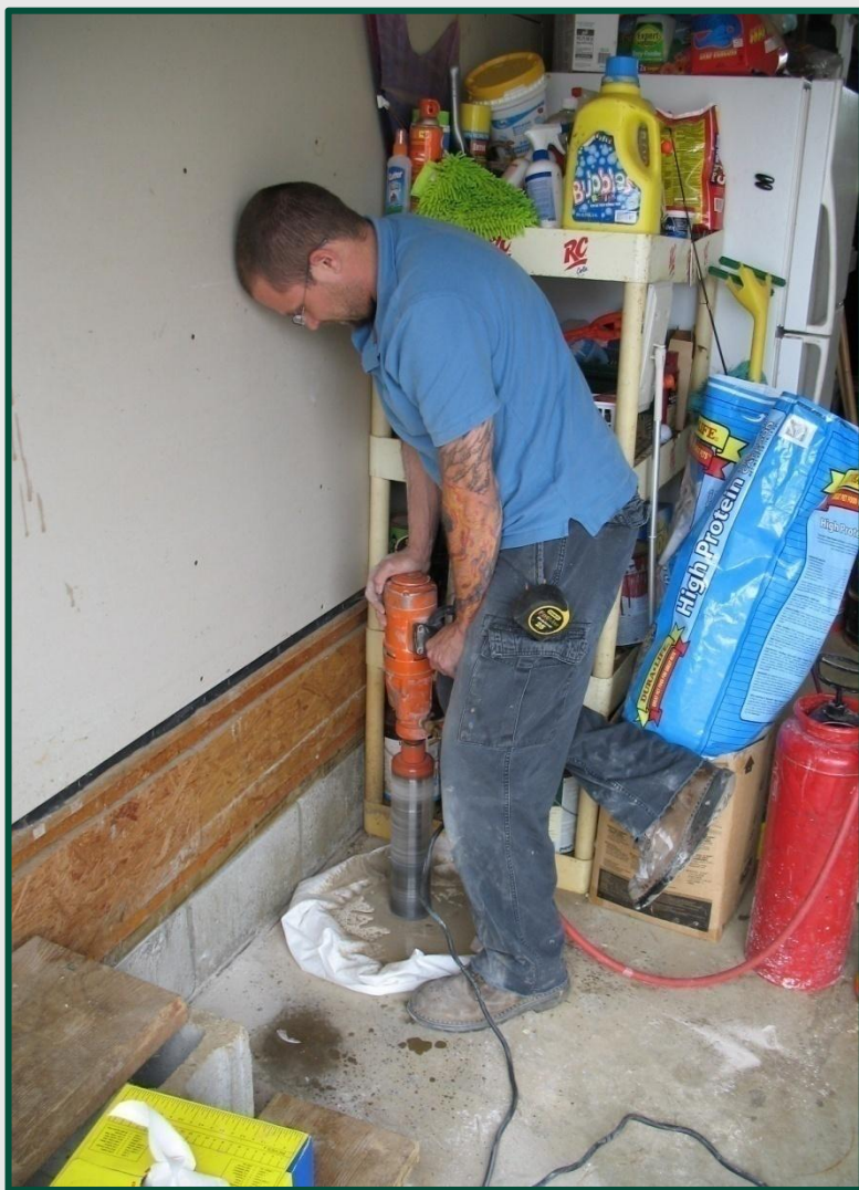
1. Core through slab
