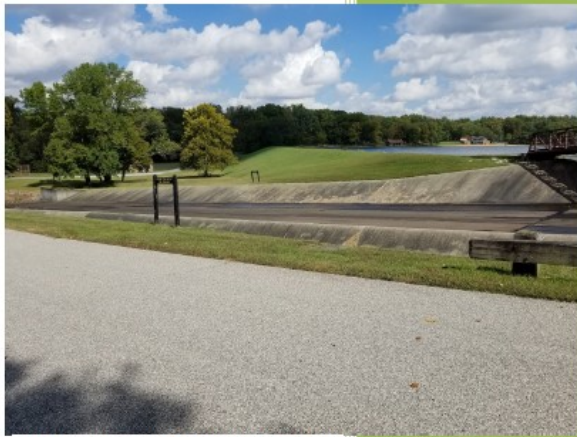
1 - Spillway, Downstream Slope, and Moon Tree in October 2018
