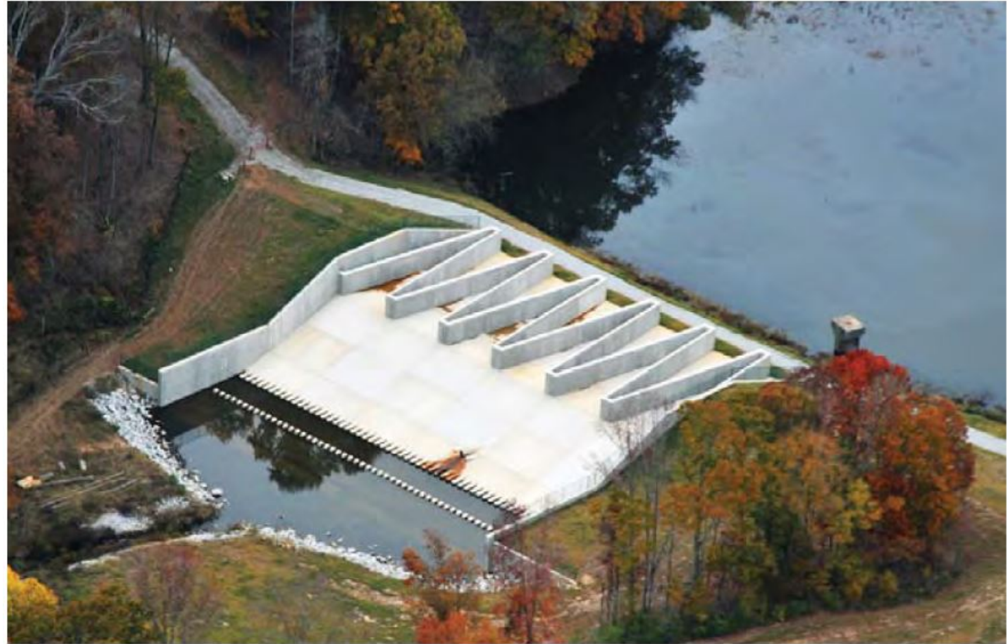
Sandy Creek 15 An aerial view of completed spillway
