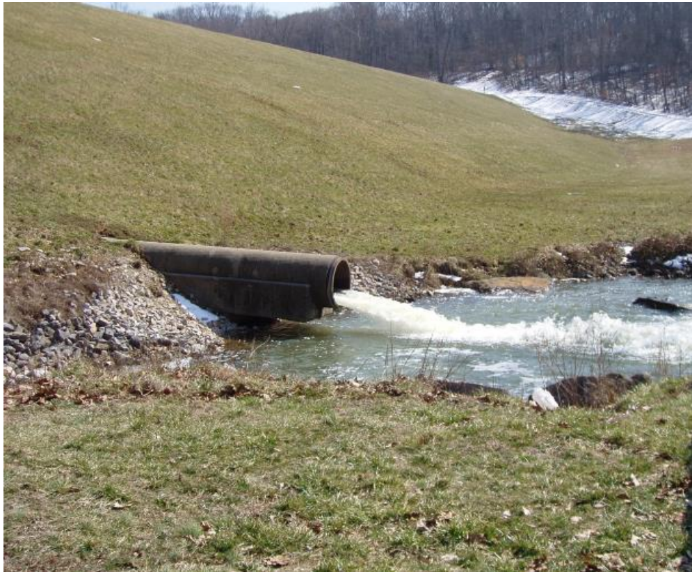
Principal Spillway Outlet Pipe
