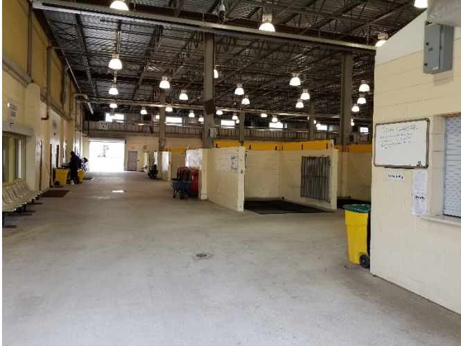
Ship-in/detention barn entrance
