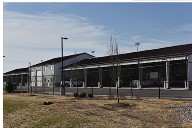
Left: Indiana Grand's brand new Track Maintenance building was erected as a part of Centaur Gaming's 2017 capital investment program. Right: The Winner's Circle in Downtown Indianapolis installed a brand new building facade giving the location a refreshed street presence.
