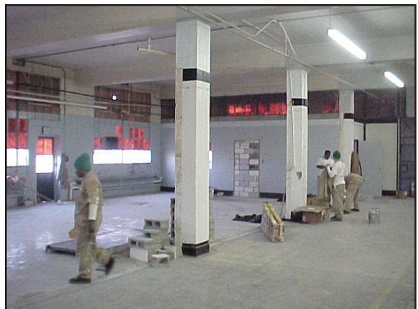
Wheels for the World shop renovation at Pendleton.
