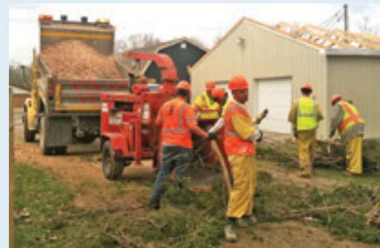
Offenders from the Henryville Correctional Facility assist Indiana Department of Transportation Crews clean up debris from a tornado that severely damaged the town of Henryville.
