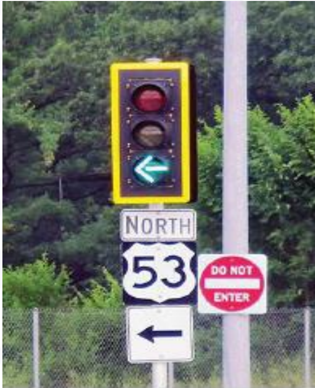
Example of a signal backplate framed with a retroreflective border.
