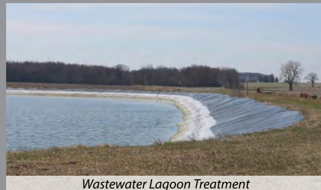
Wastewater Lagoon Treatment
