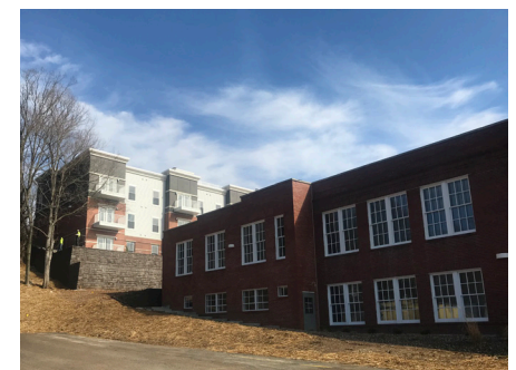
Corydon School Senior Lofts Construction Progress
