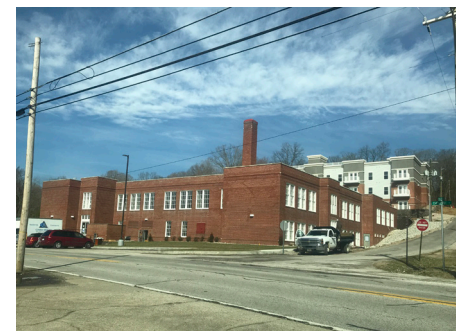
Corydon School Senior Lofts Construction Progress
