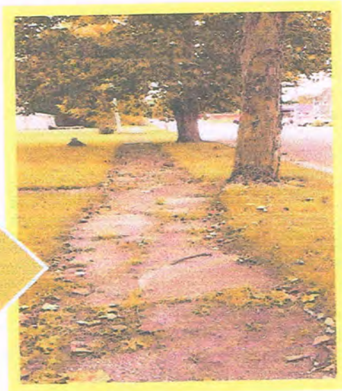
East Main St.
