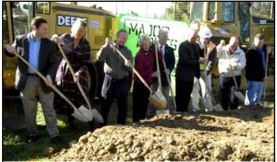
Governor Daniels joins the Indiana Department of Transportation and local elected officials for a groundbreaking event celebrating the beginning of the State Road 261 expansion project.
