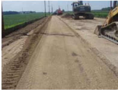
The latest project to use tire shreds as an alternative fill is pictured. This view is southbound on SR 19 in Kosciusko County.
